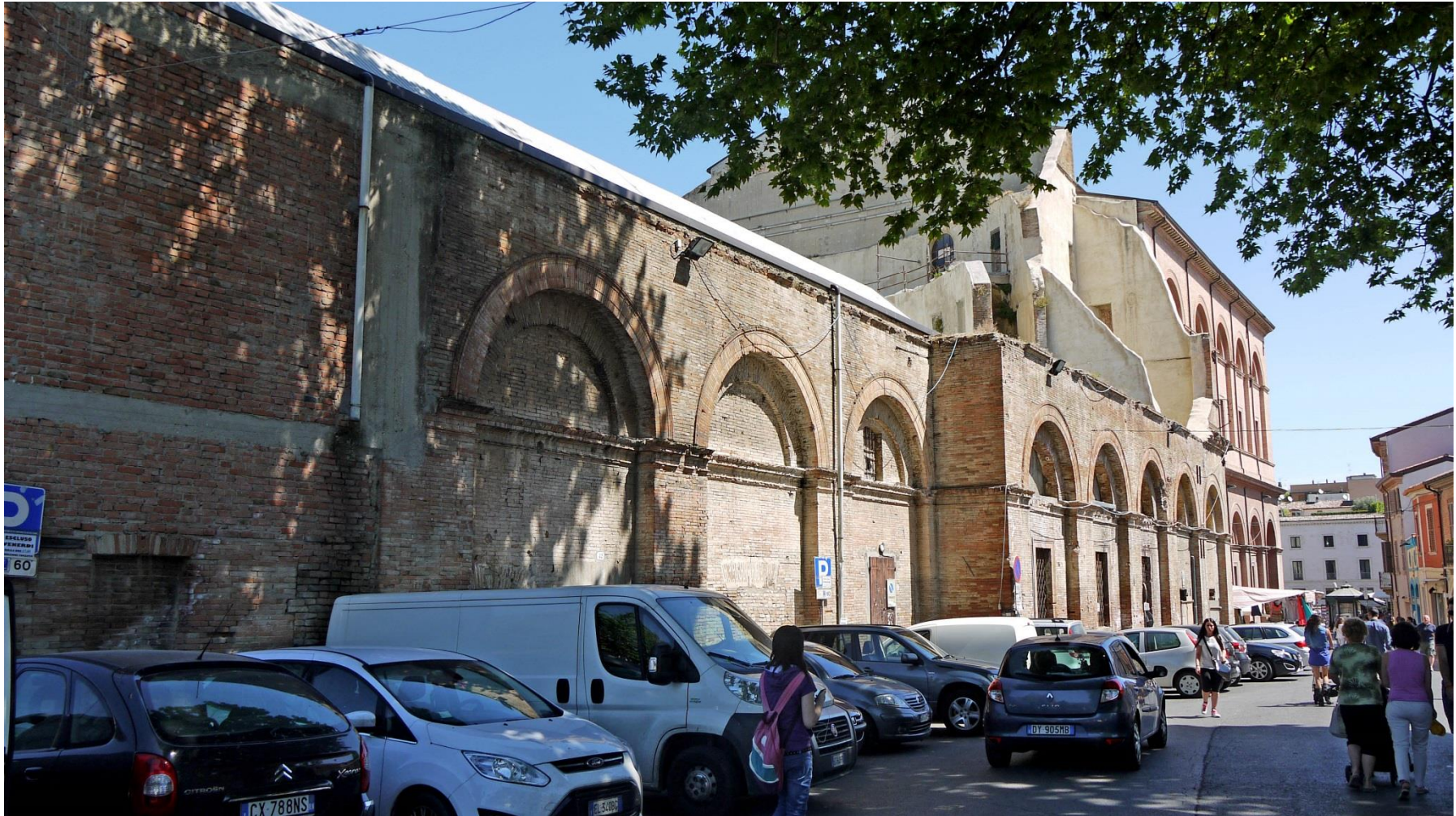
Translating wall via Poletti side
